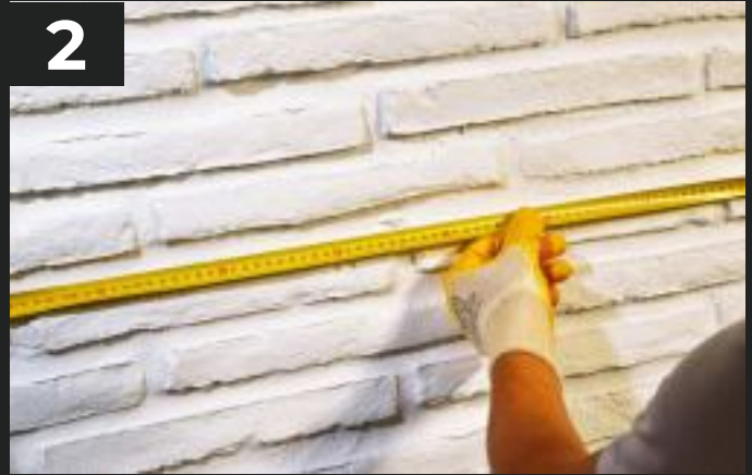
2. Anzubringendes Panel ausmessen Scaling of the panel to be applied
